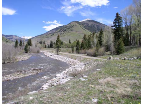
Figure 2-5: This section of the channel is not natural and has been “engineered” to be stable during a flood event. However, this alteration often propagates instability downstream.
