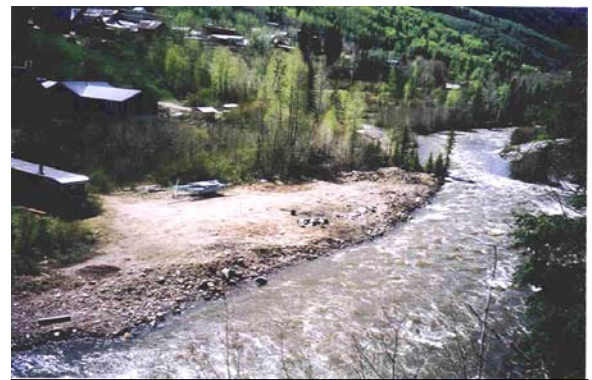
Figure 2-6: All stabilizing riparian vegetation has been removed in front of this development.
