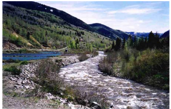
Figure 2-9: View downstream toward Rico along the Dolores River. The St. Louis settling ponds (left) are isolated from the river by lining the channel bank with riprap.
