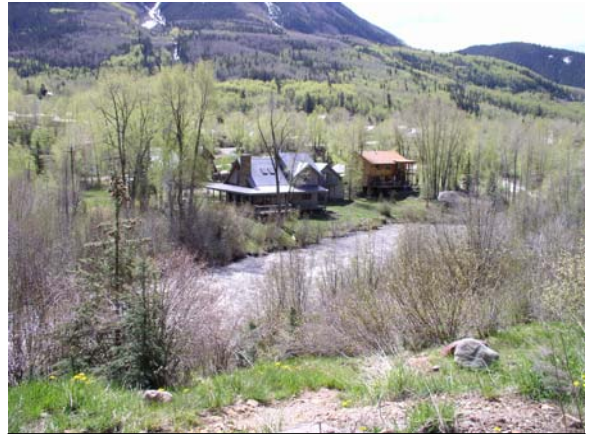
Figure 2-7: Several residential structures have been constructed within the river floodplain.
