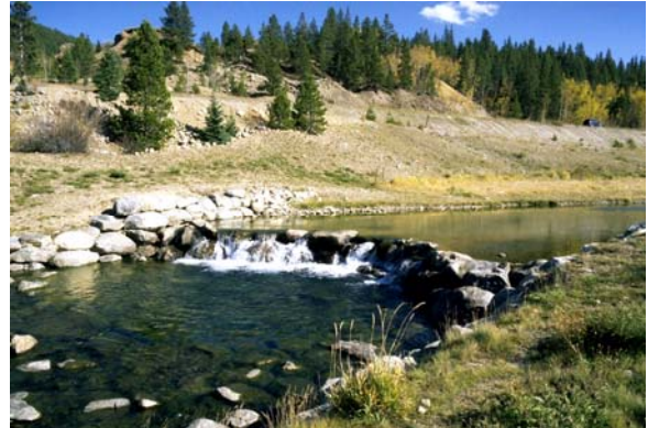
Boulder drop structure on the Blue River, Colorado.
