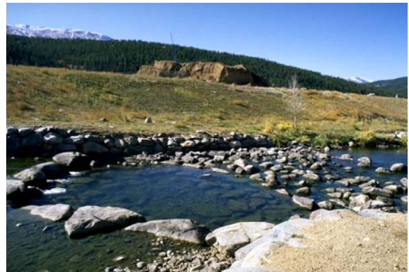
This picture of a drop structure on the Blue River near Breckenridge shows the primary upstream drop and the downstream control drop which forms the plunge pool.
